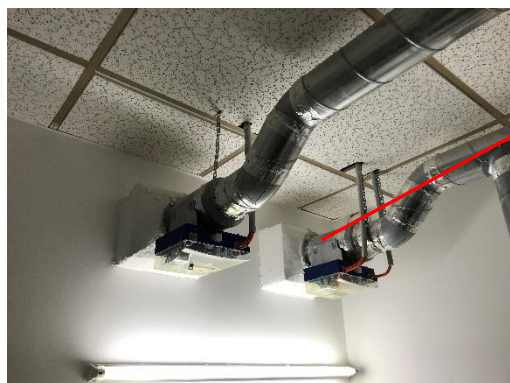
Gaine clapet VMC
